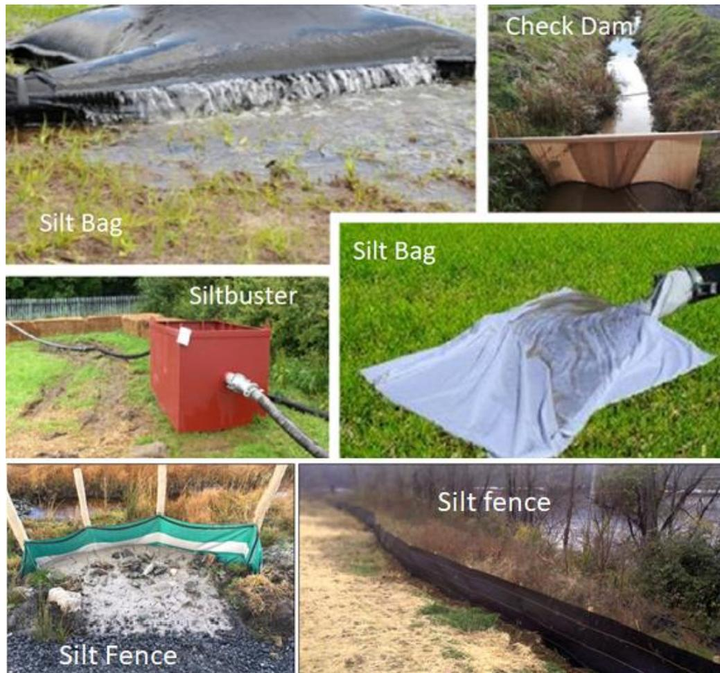
Figure 2-5: Examples of Proprietary Silt Control measure Trench Drainage
